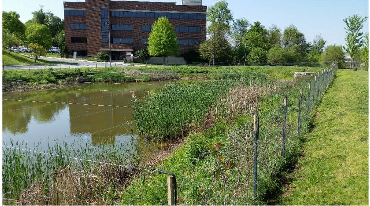
Goose Barrier at Xfinity Center Stormwater Pond
