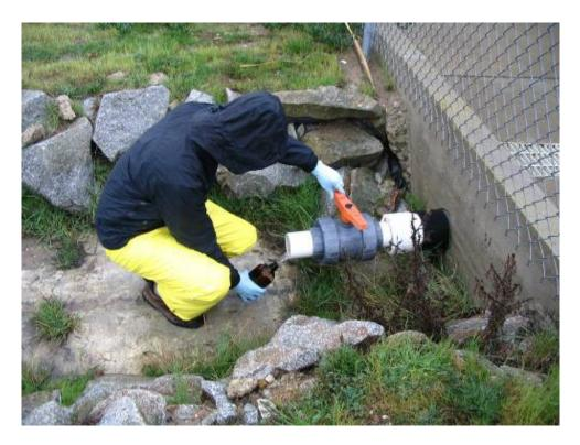
Figure 1. Stormwater discharges to the slot drain and is conveyed offsite through a valved pipe.
