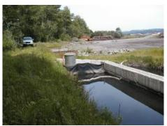
Figure 5. Outlet discharging from detention pond.
