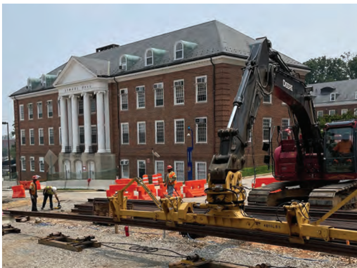
Construction impacts Campus Drive
