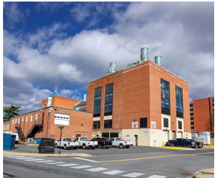
The campus Combined Heat and Power plant.
