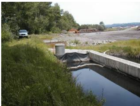
Figure 5. Outlet discharging from detention pond.
