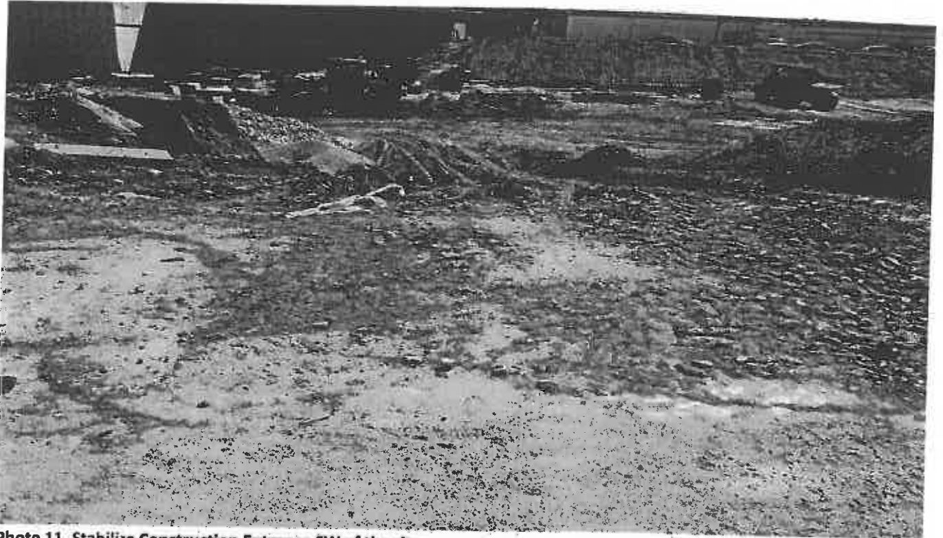
Photo 11. Stabilize Construction Entrance SW of the site
