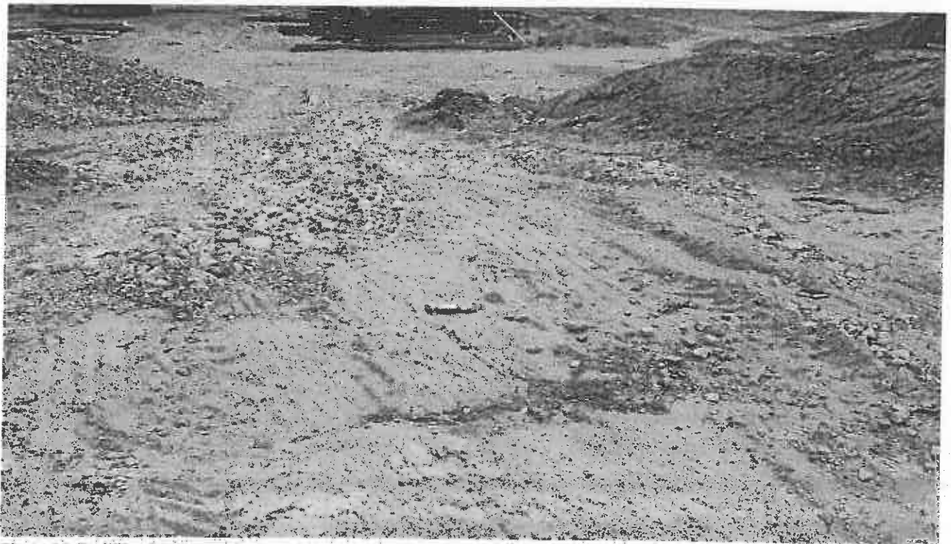
Photo 14. Stabilized Construction Entrance on Cole Fieldhouse Drive NE of the site
