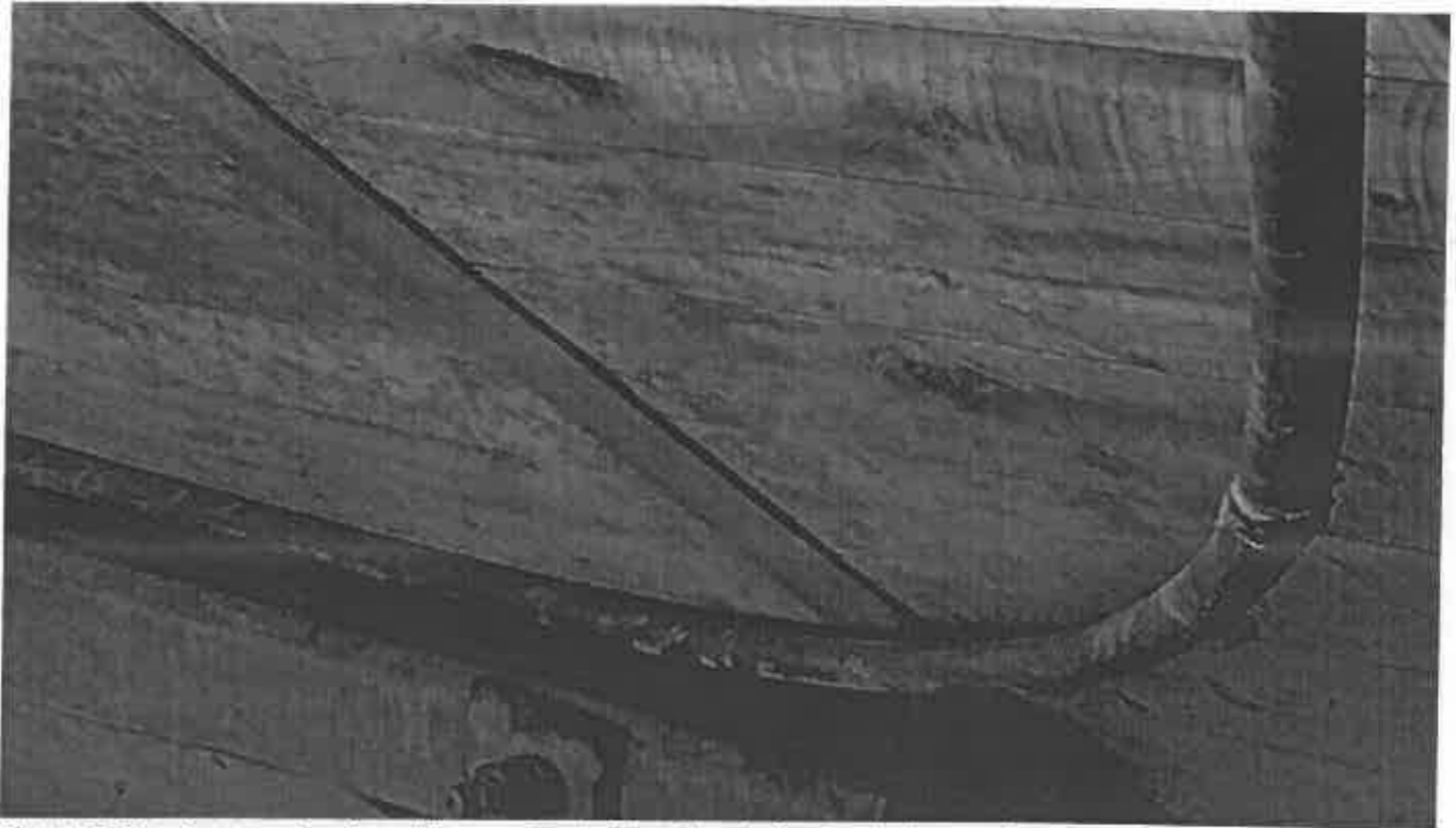
Photo 15. Ongoing pumping of muddy groundwater from foundation footing into active stormdrain onsite.
