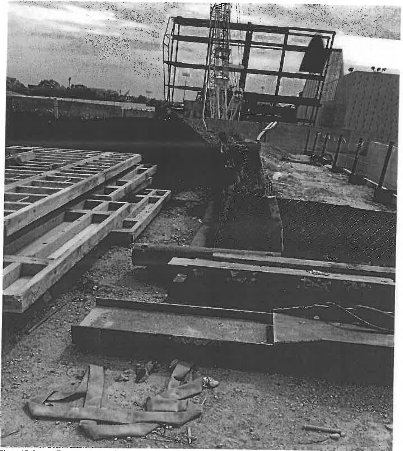
Photo 15. Super Silt Fence SW of the site
