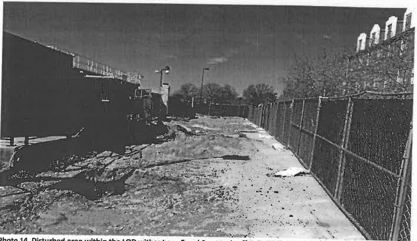
Photo 14. Disturbed area within the LOD without any E and S controls off Cole Fieldhouse Drive NW of the site
