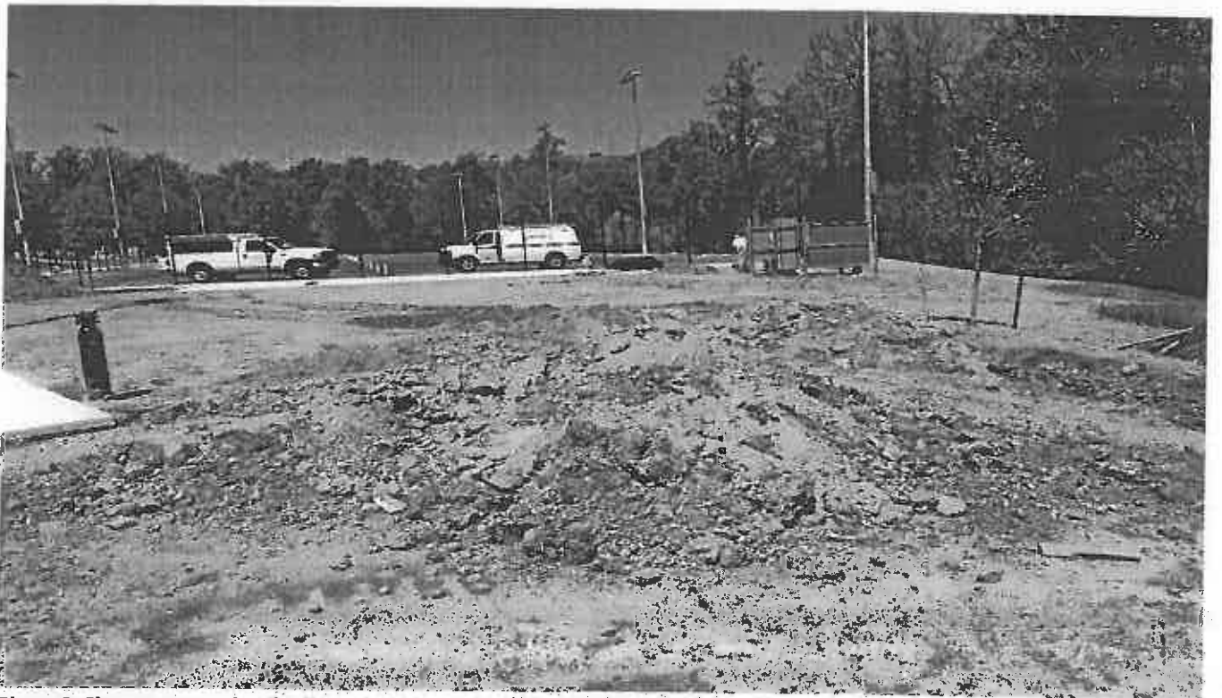
Photo 2. Shows exposed soil adjacent storm water management pond at the new tennis court
