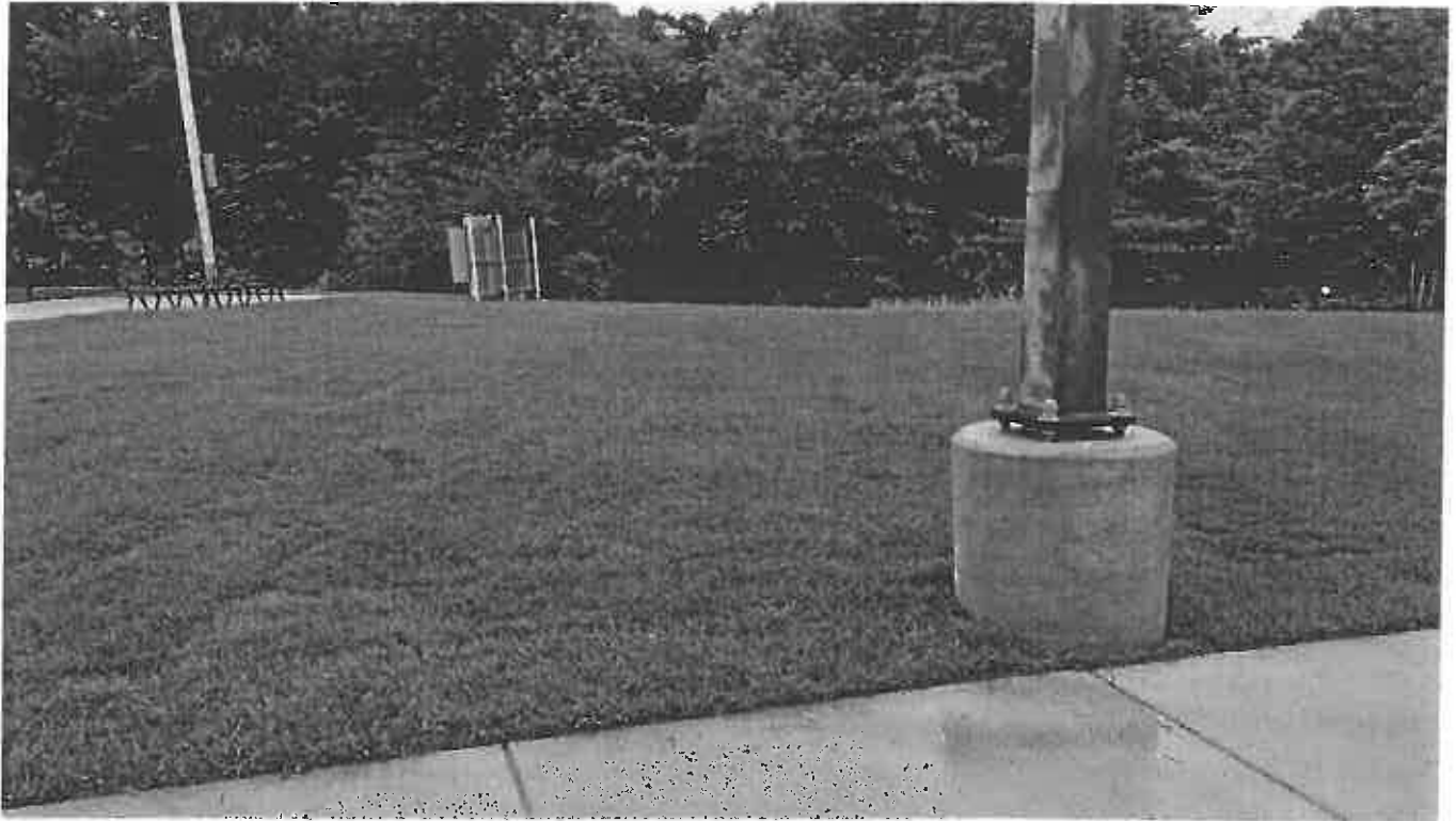
Photo 1. Shows sod stabilization adjacent the storm water management pond at the new tennis court
