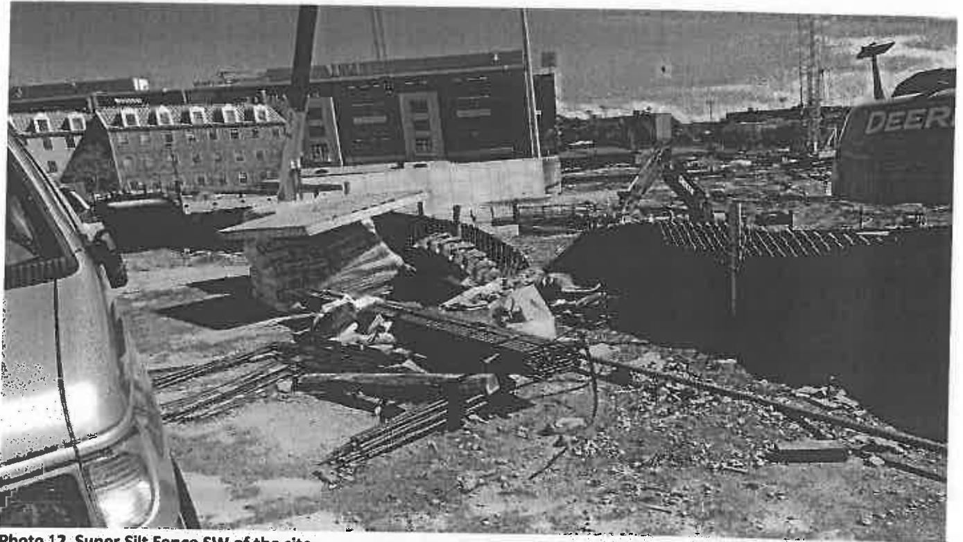
Photo 12. Super Silt Fence SW of the site
