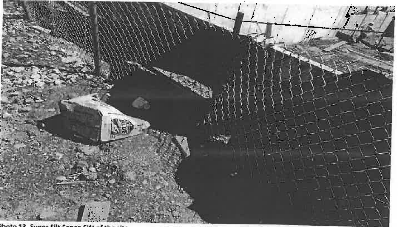
Photo 13. Super Silt Fence SW of the site
