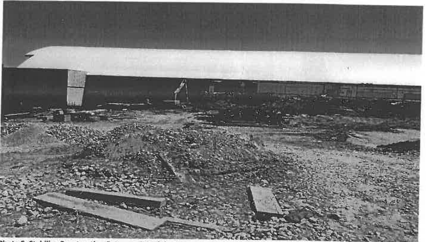
Photo 5. Stabilize Construction Entrance SW of the site
