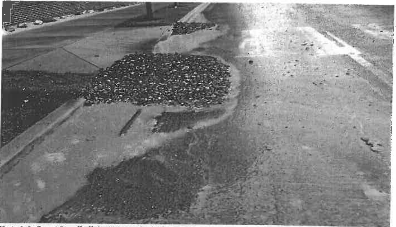
Photo 1. Sediment Runoff off site NW on Cole Fieldhouse Drive.
