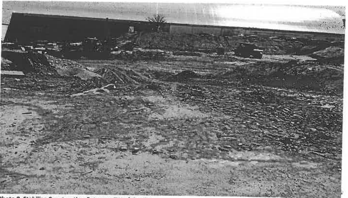
Photo 9. Stabilize Construction Entrance SW of the site
