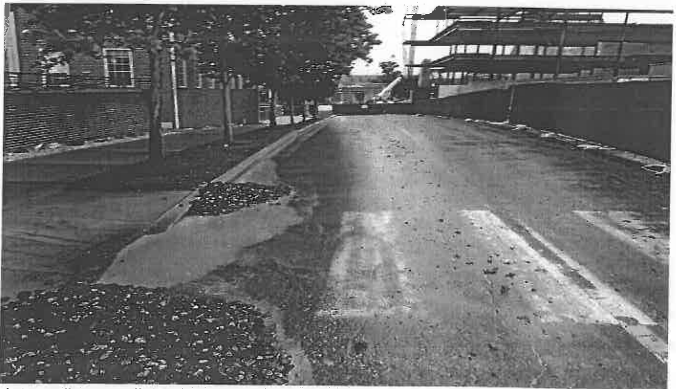
Photo 2. Sediment Runoff off site NW on Cole Fieldhouse Drive.
