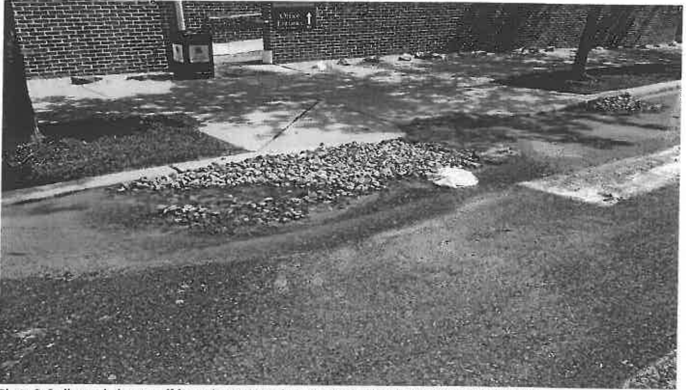
Photo 9. Sediment laden runoff from site to stormdrain on Cole Field Drive in photo 1 off the site.
