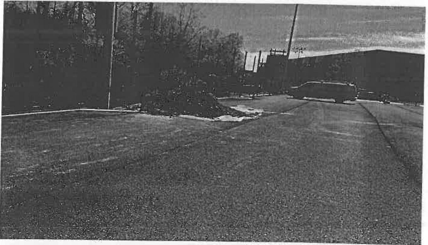
Photo 8. Sediment placed on paved surface at the new tennis court with potentials to impact the stormdrain
