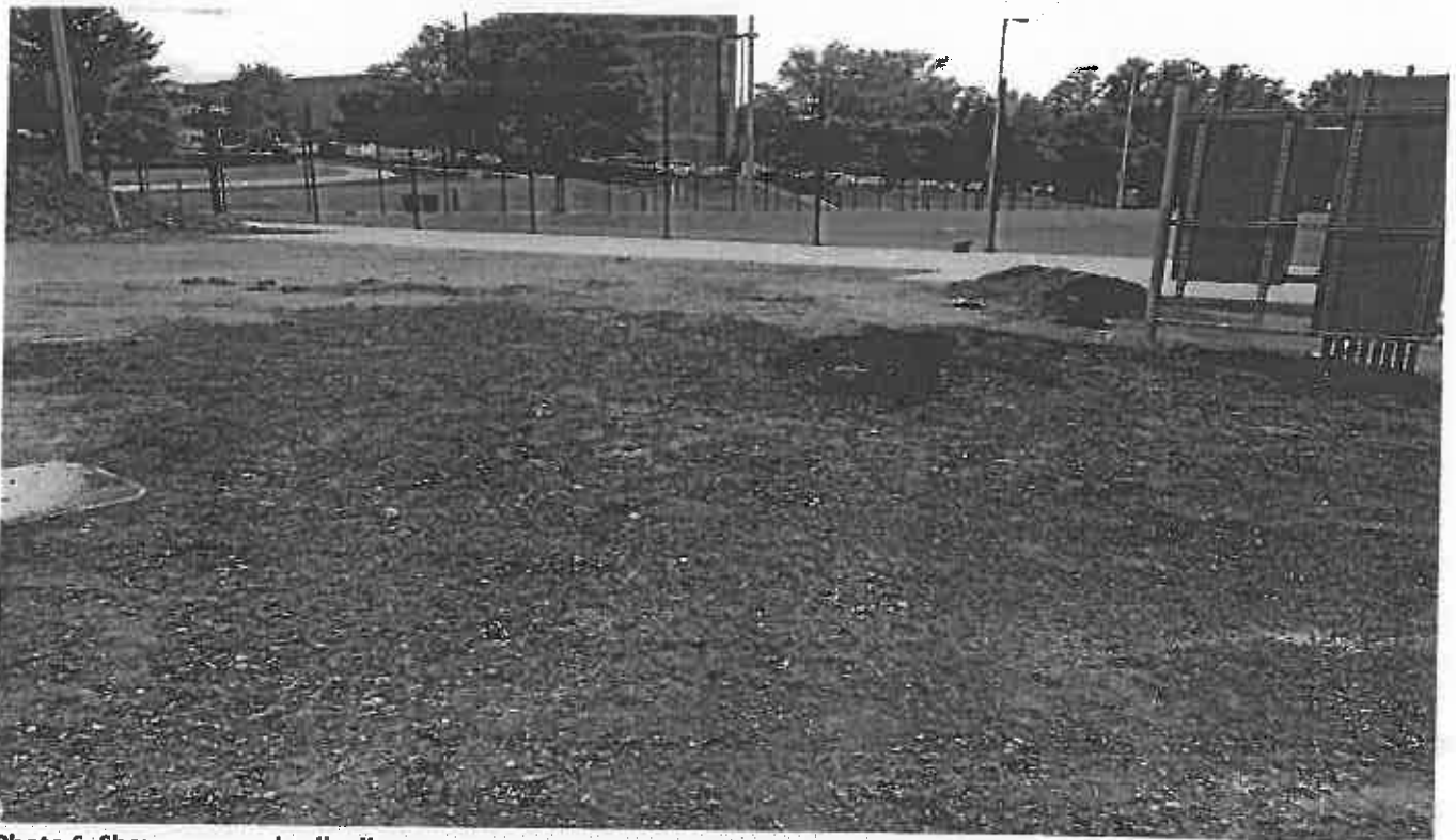
Photo 6. Shows exposed soil adjacent storm water management pond at the new tennis court
