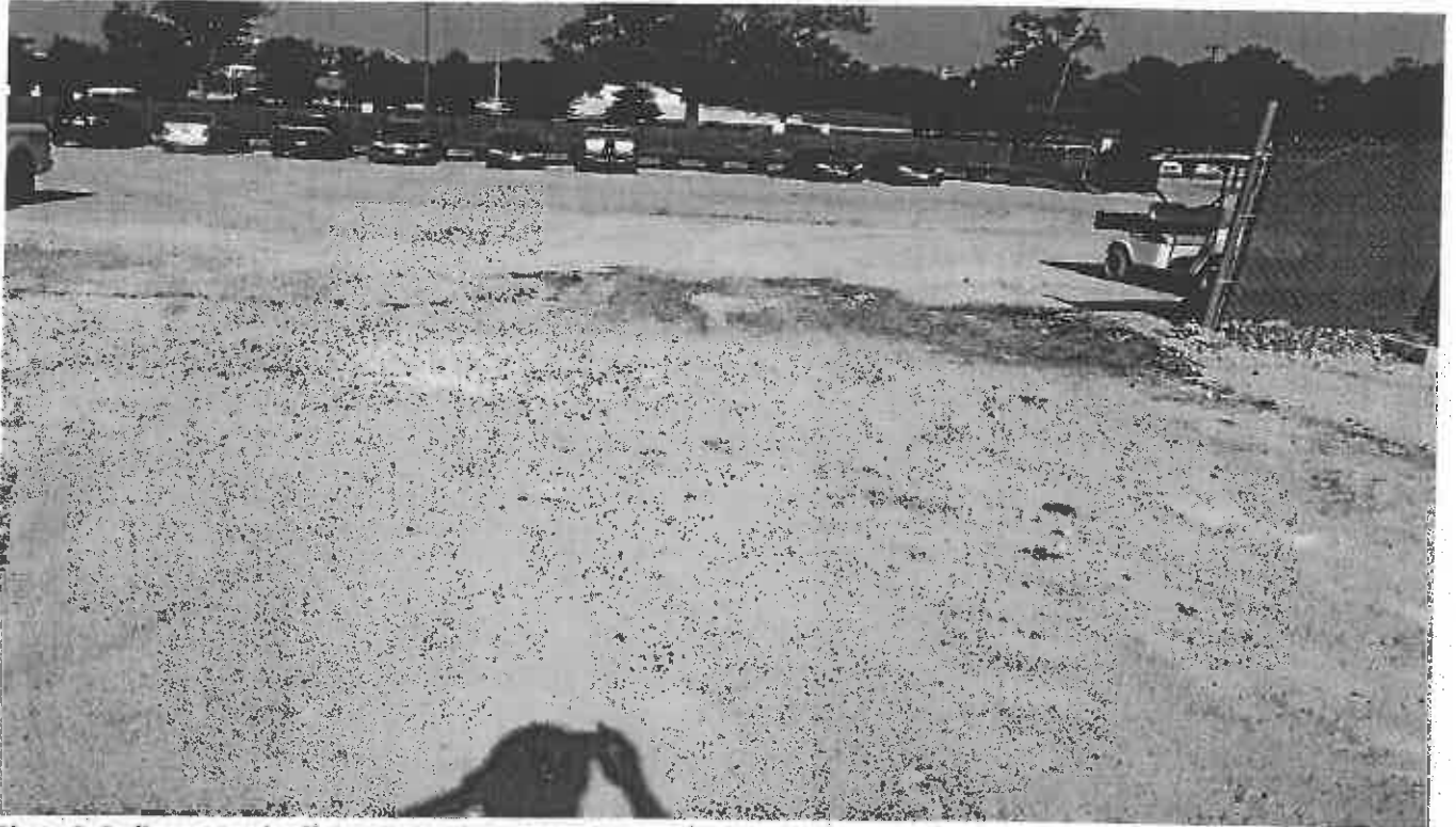
Photo 9. Sediment track off the site to the parking lot South of the site
