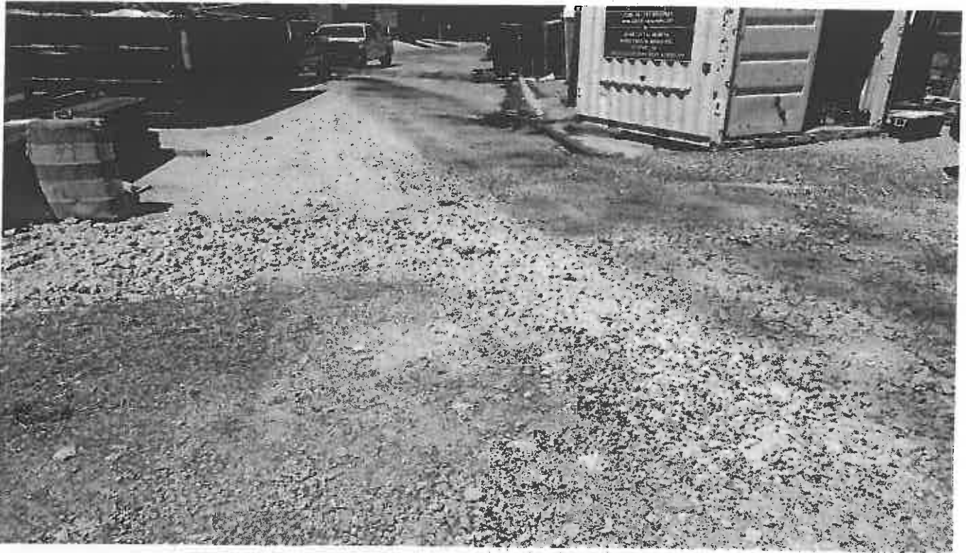
Photo 15. Stabilized Construction Entrance on Cole Fieldhouse Drive NW of the site
