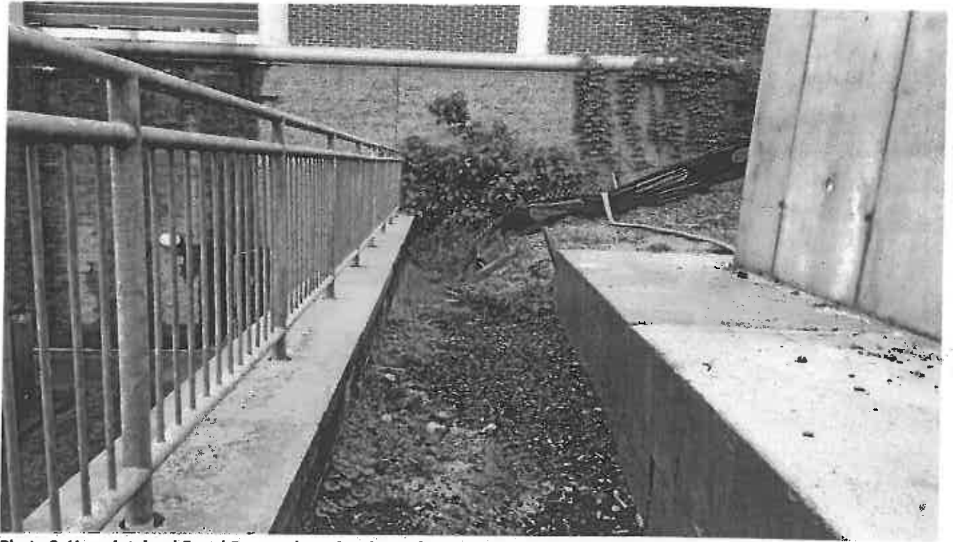
Photo 9. Unmaintained E and S controls at the Slope of the Tunnel Project North of the Site
