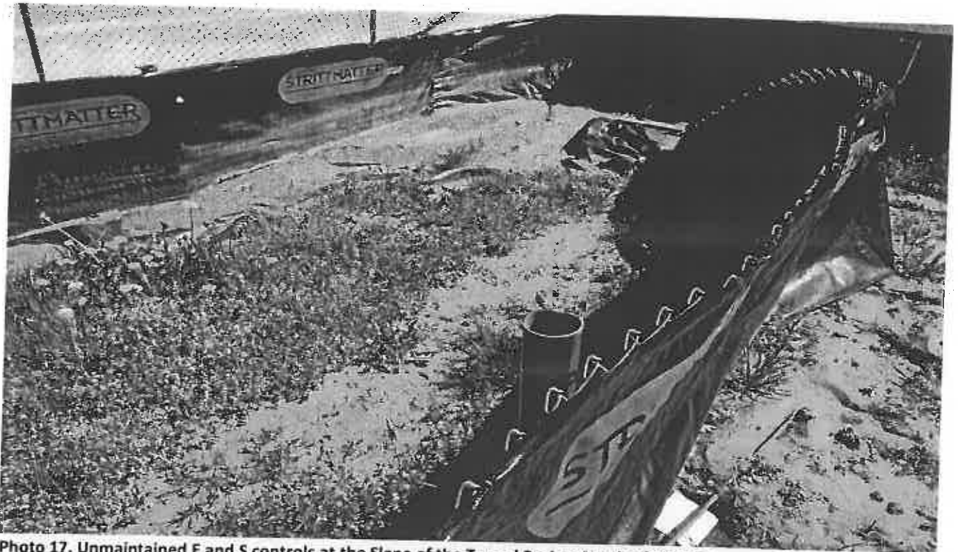
Photo 17. Unmaintained E and S controls at the Slope of the Tunnel Project North of the Site
