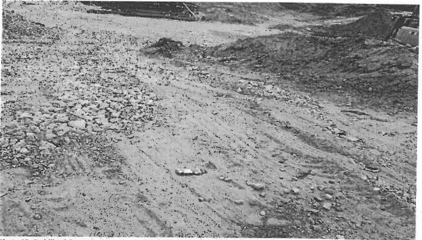
Photo 13. Stabilized Construction Entrance on Cole Fieldhouse Drive NE of the site
