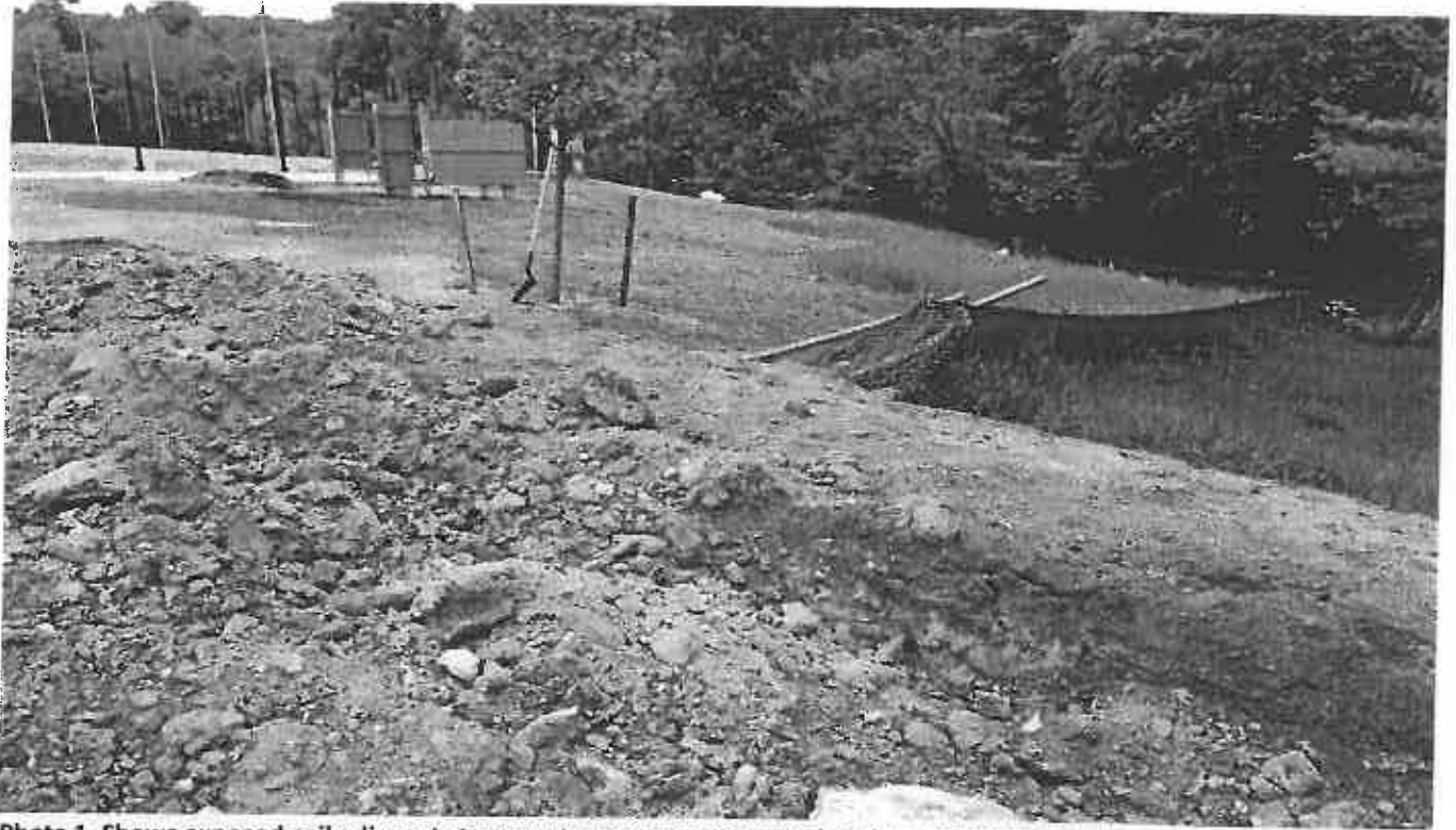
Photo 1. Shows exposed soil adjacent storm water management pond at the new tennis court
