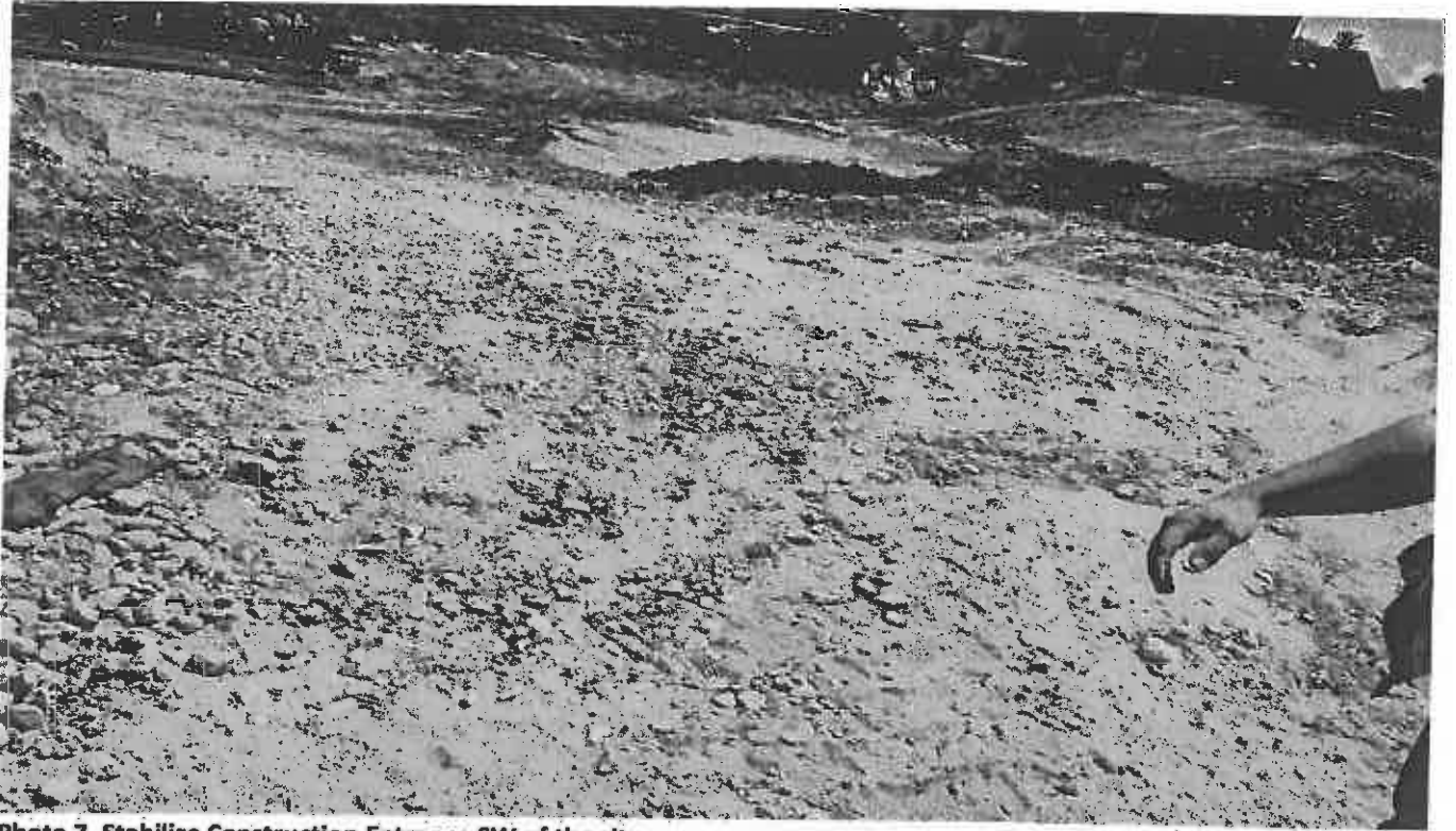
Photo 7. Stabilize Construction Entrance SW of the site
