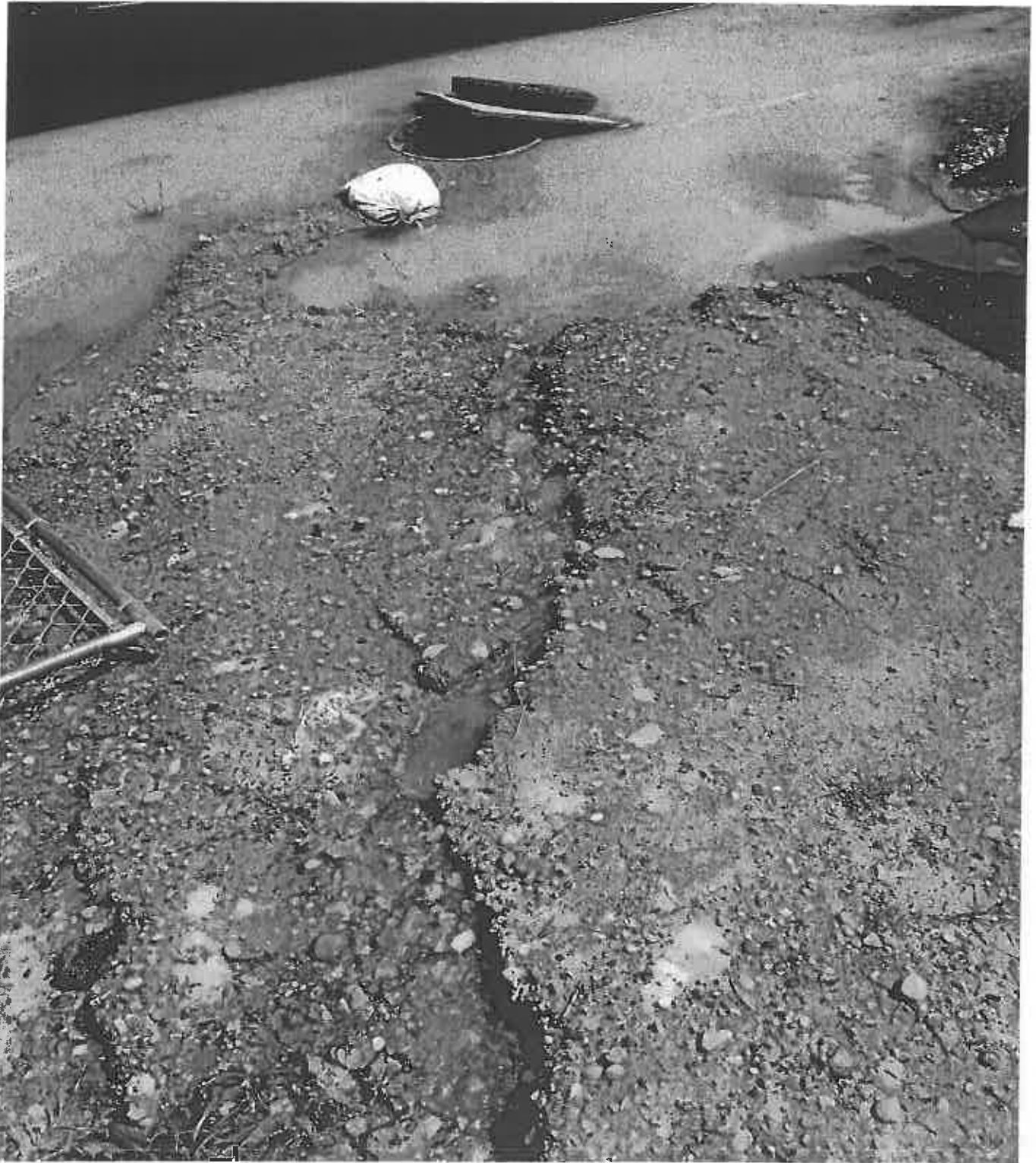
Photo 5. Sediment filter bag placed on exposed soil NW of the site near the sediment tank going into stormdrain
