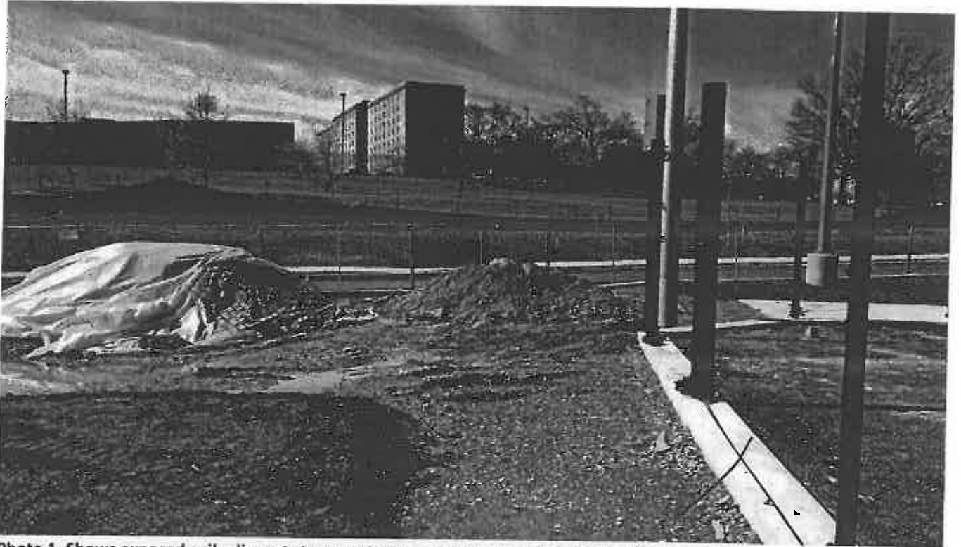
Photo 1. Shows exposed soil adjacent storm water management pond at the new tennis court
