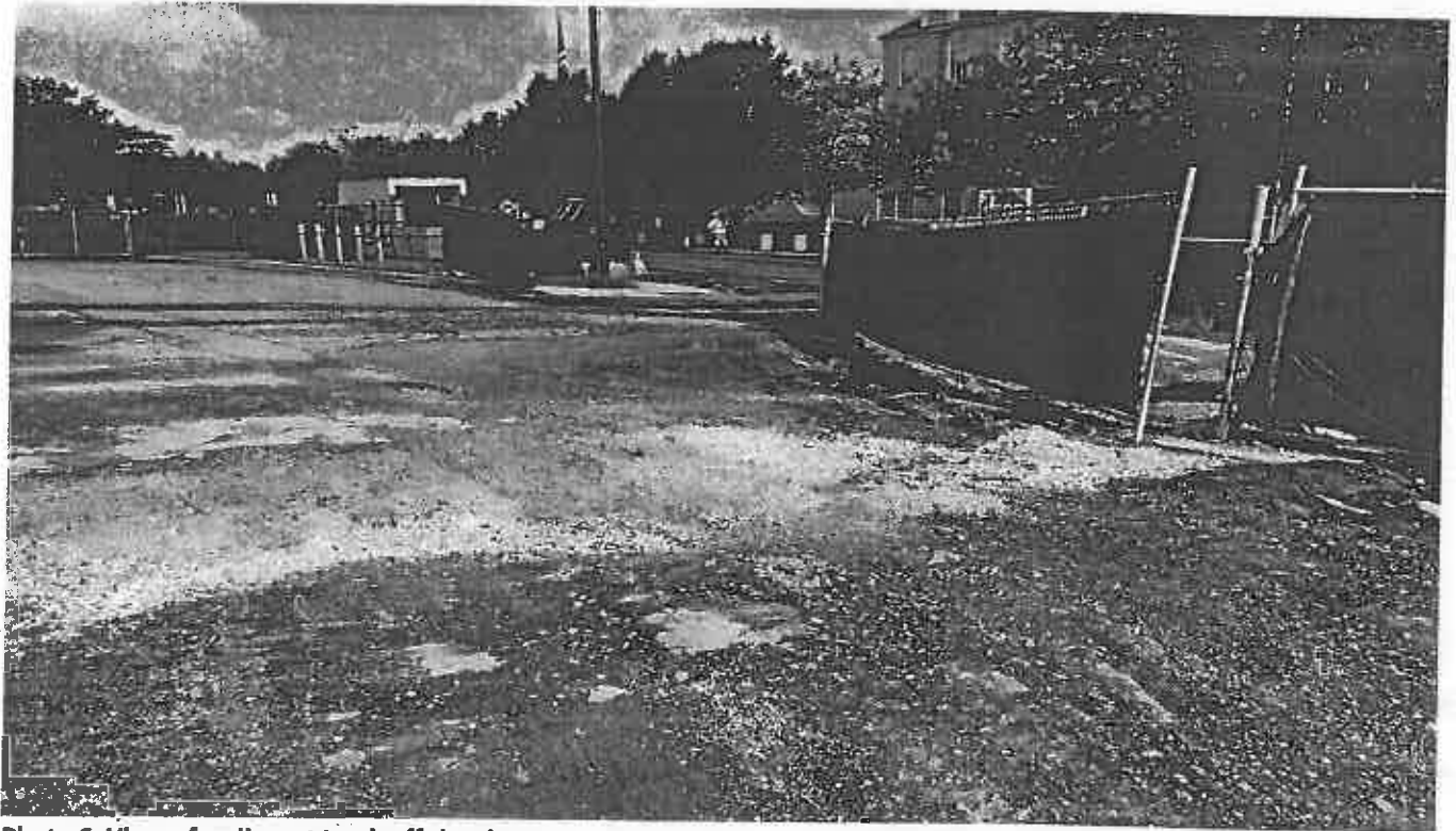
Photo 6. View of sediment track off the site
