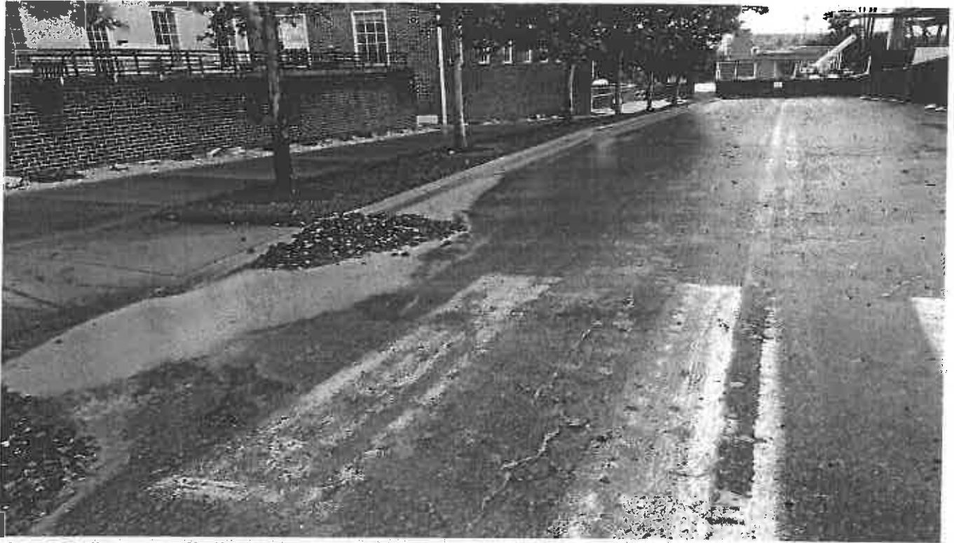
Photo 3. Sediment Runoff off site NW on Cole Fieldhouse Drive.
