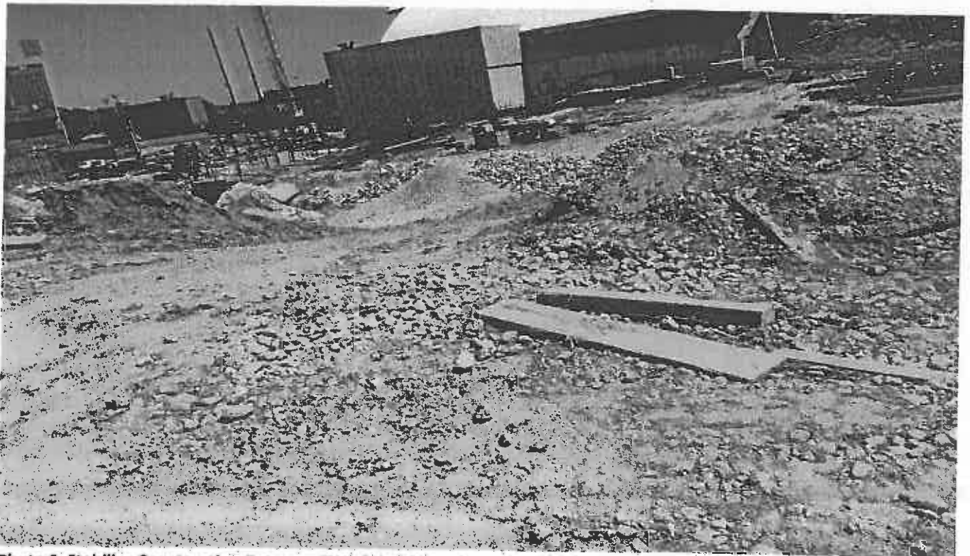
Photo 6. Stabilize Construction Entrance SW of the site
