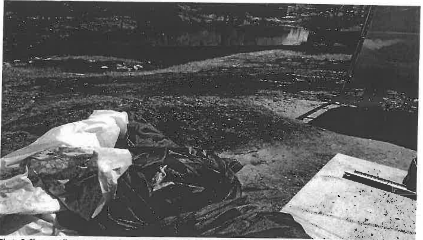
Photo 3. Shows sediment saturated storm water management pond at the new tennis Court.
