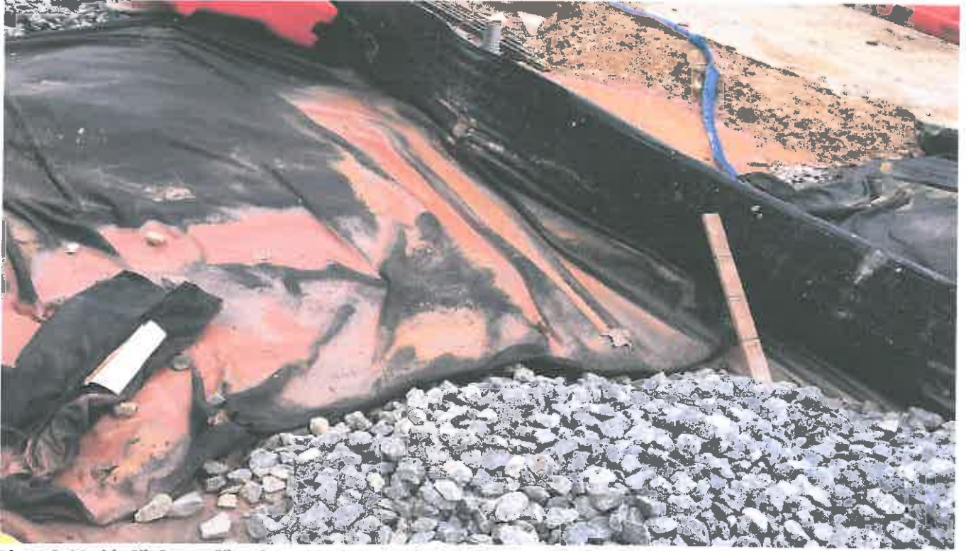
Photo 3. Muddy Silt Bag or Filter Bag with Close Proximity to the Stormdrain
