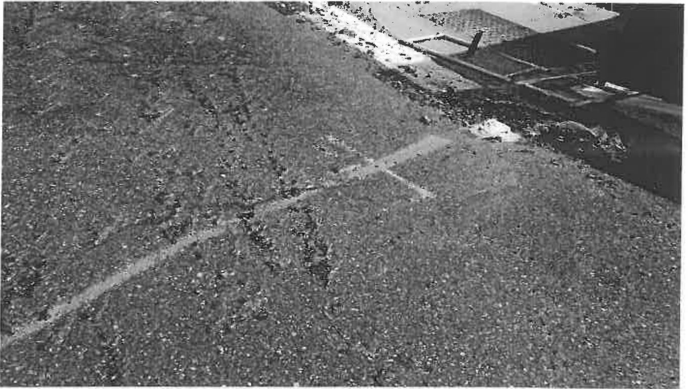
Photo 7. Sediment laden runoff from site to stormdrain on Cole Field Drive in photo 1 off the site.
