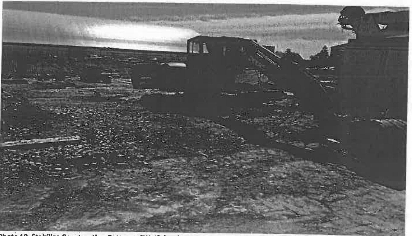
Photo 10. Stabilize Construction Entrance SW of the site
