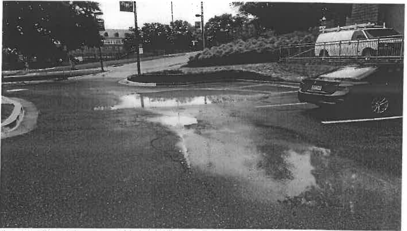
Photo 13. Sediment laden stormwater runoff from site to the stormdrain at Gossett Football Team House lot.
