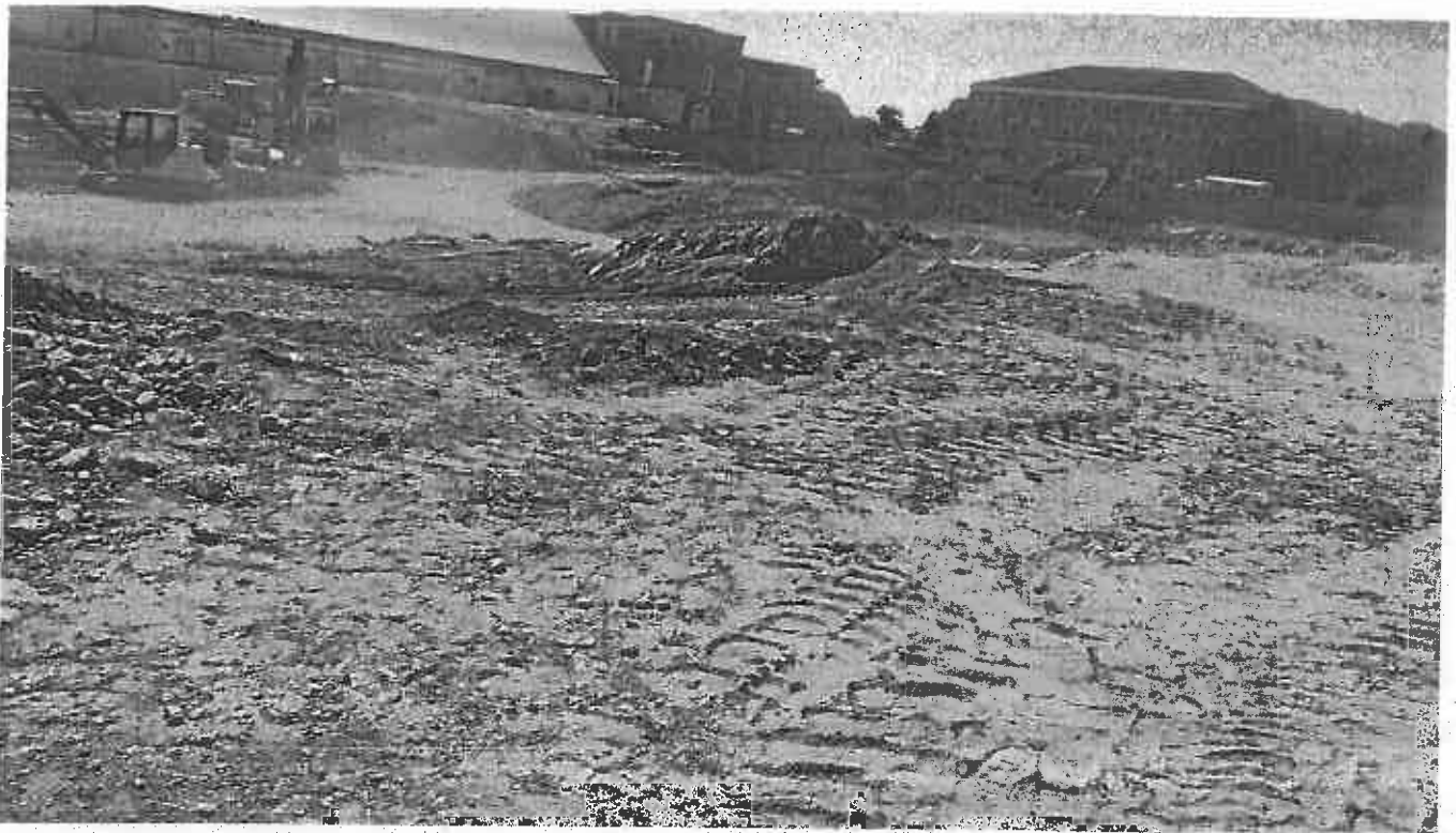
Photo 2. Stabilize Construction Entrance without aggregate stones tracking mud on paved road SW site of site
