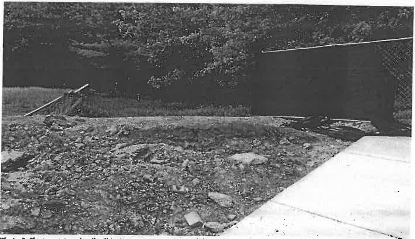
Photo 2. Shows exposed soil adjacent storm water management pond at the new tennis court
