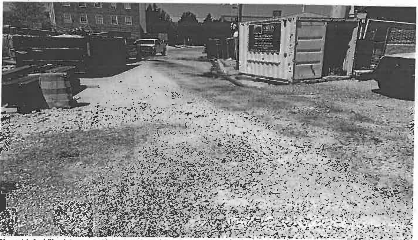
Photo 14. Stabilized Construction Entrance on Cole Fieldhouse Drive NW of the site
