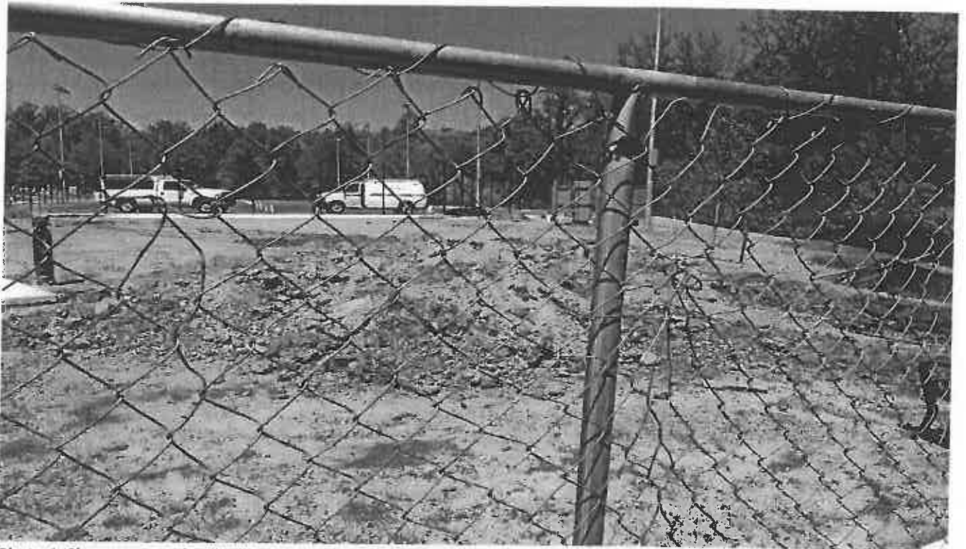
Photo 1. Shows exposed soil adjacent storm water management pond at the new tennis court
