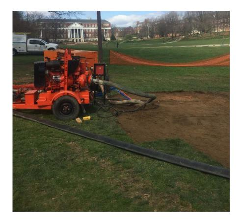
Top: looking northwest from Woods Hall, the ground cover that contacted biosolids was treated with lime to a pH of 12 and removed for disposal. The source of the sewage overflow was excavated to make the necessary repairs.
