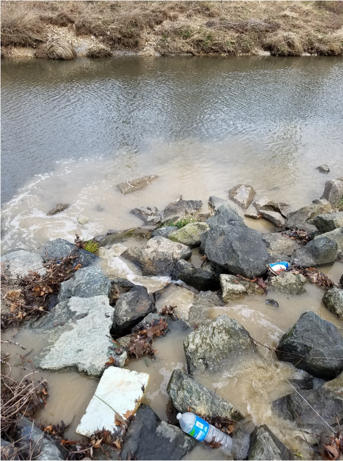
Top left: sediment laden water discharging from Outfall 003 to Paint Branch Creek.
