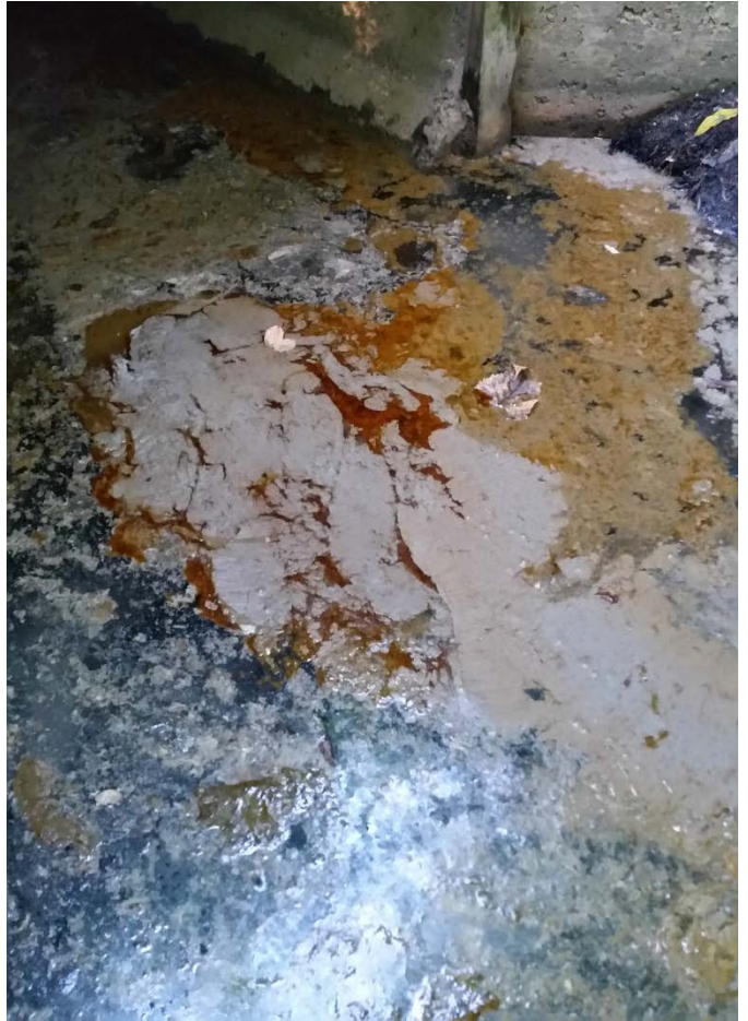
Top left: Ellicott Dining Hall loading dock with food oil/grease leaking from compost compactor Top right: Food oil/grease on water surface at Outfall 019 Bottom: Ellicott Dining Hall loading dock with food oil/grease leaking from compost compactor
