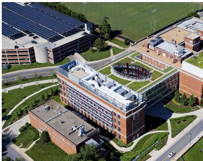
Green Roof - Physical Sciences Building
