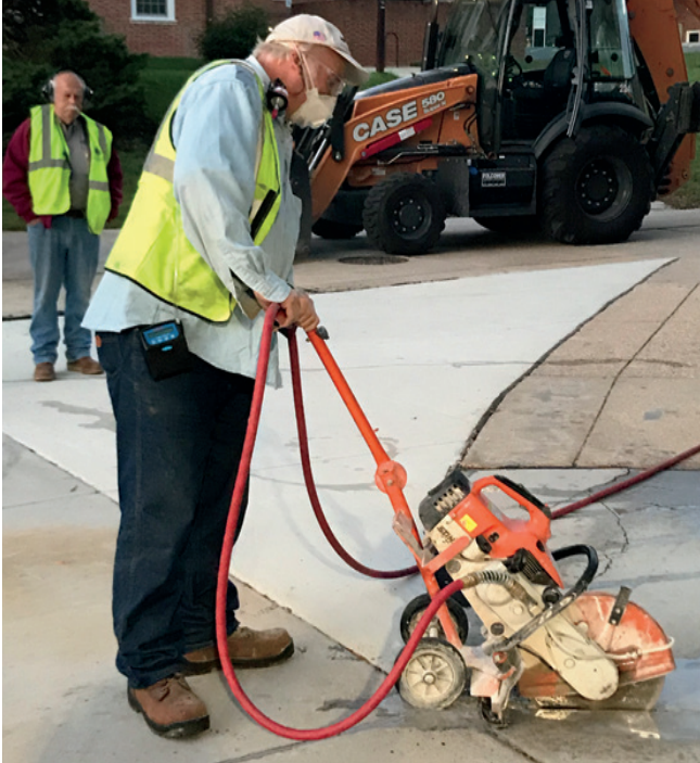
A Facilities Management staff member cuts concrete.
