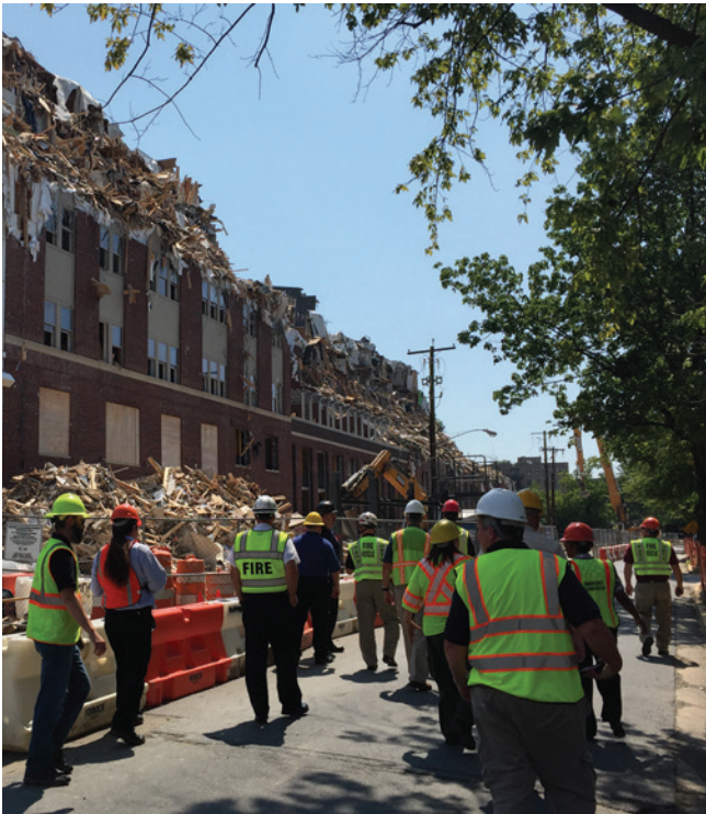
Maryland Fire Marshals Committee members at site of Fuse 47 fire.
