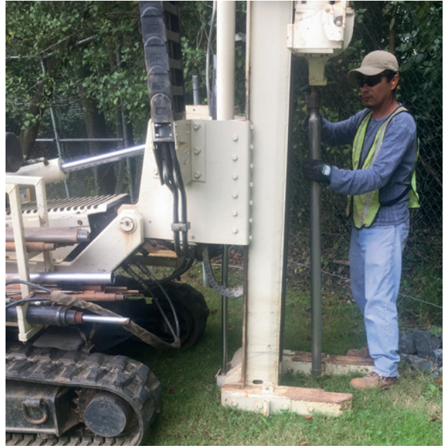
Geoprobe sampling of soil and groundwater.
