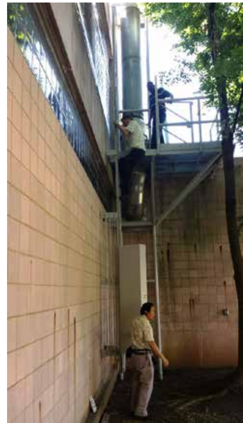
Passive fall protection at Animal Science.
